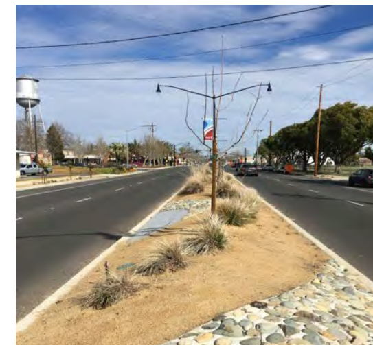
Bridge Street - Median Improvements
