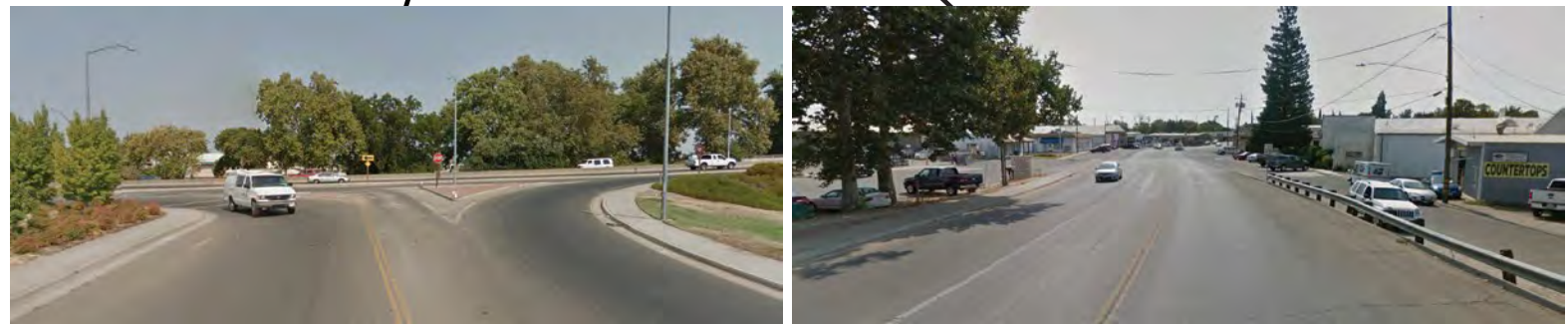
SR 20 - SUTTER STREET AND FEATHER RIVER BRIDGE ENTRY
