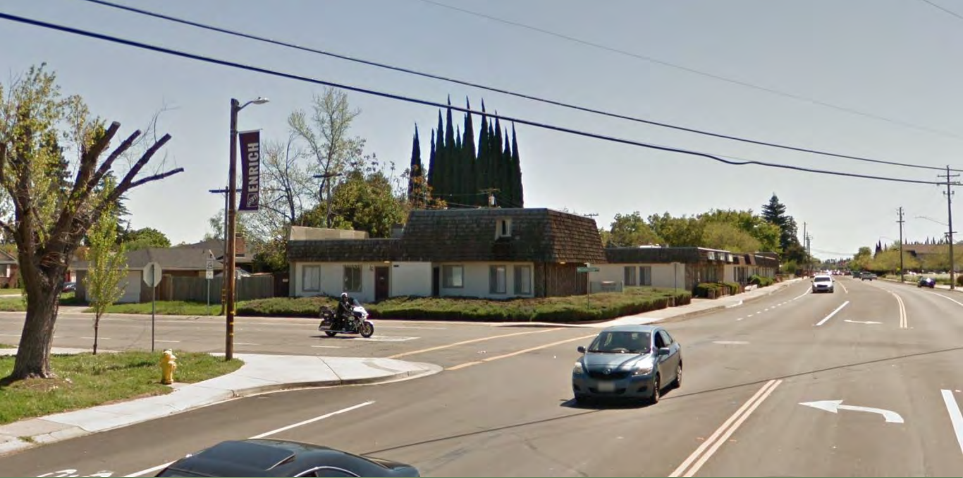
North Area – Stabler Ln. and Grey Ave.
