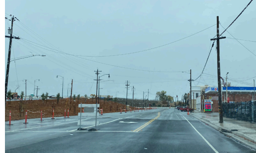
Road Construction Near the River
