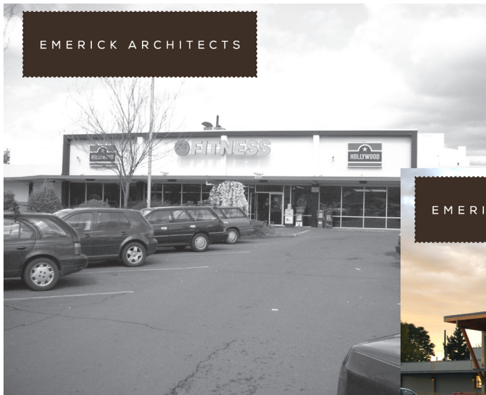
BEFORE: Dated Box Last Used as a Gym
