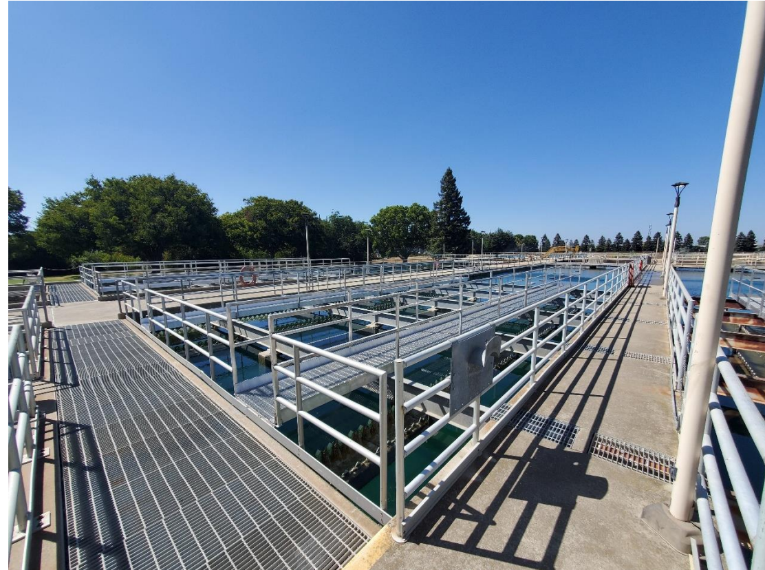
WTP – Catwalks over Sedimentation Basins
