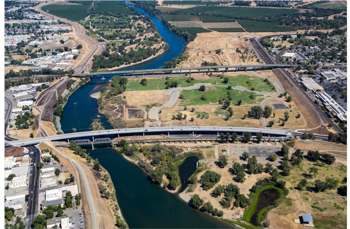
Fifth Street Bridge Replacement
