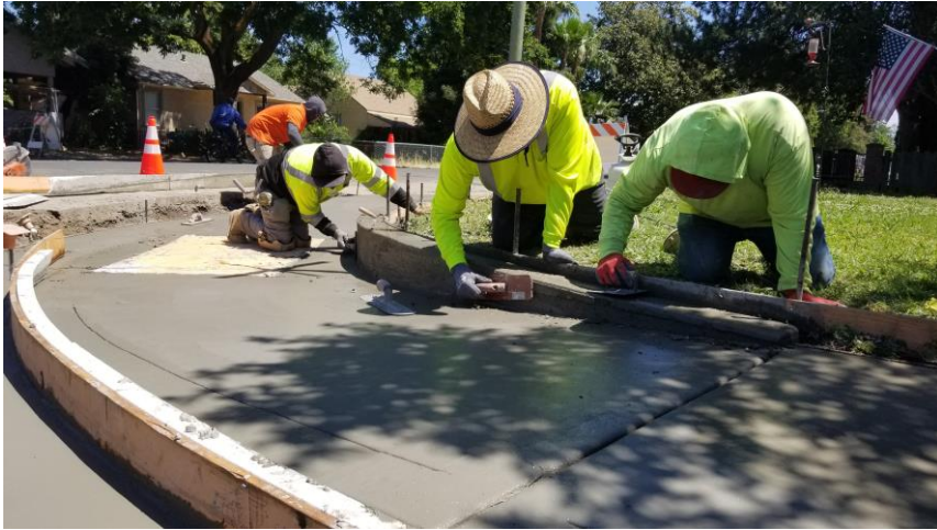
ADA Improvements Project
