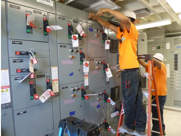
New Control Panels
