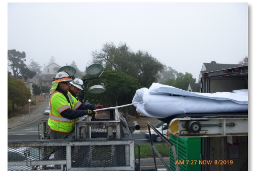
Mare Island CIPP Rehab
