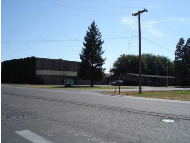
Existing private school located on Harding Road
