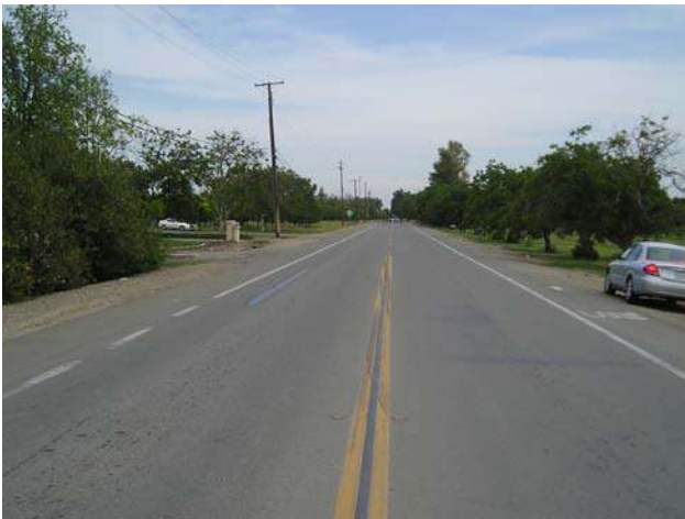
Existing street segment of Lincoln Road
