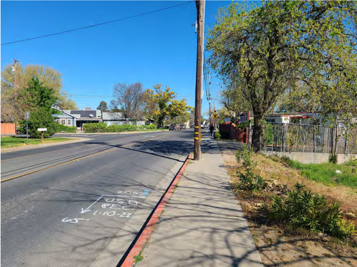
Figure 6: Intersection of Del Norte Avenue and Market Street
