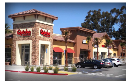
Commercial development representative of the Neighborhood Commercial category.
