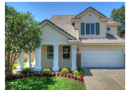
Articulate roof form through use of dormers, porch roofs to avoid monolithic appearance.
