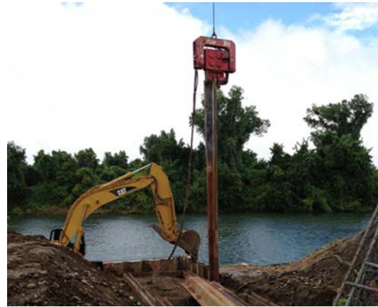
Installing Shoring for the 54" Line
